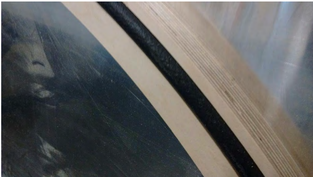
Figure 14: Rubber gasket, embedded into the frame.
